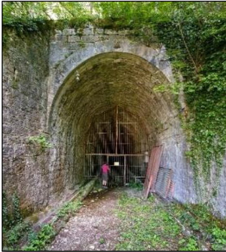
Tunnel de la station OG35 (Ain)
